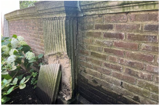
Figure 17. Spalled limestone pilaster in the west courtyard.
