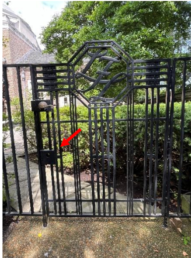
Figure 6. Existing appearance of the gate. When the masonry walls were lowered in height, the gates were trimmed at the top and bottom to fit the altered opening. The latch handle was relocated to a new location; the arrow indicates the original latch box.
