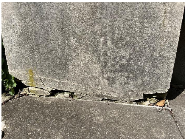
Figure 21. Spalled limestone at the base of a pier.
