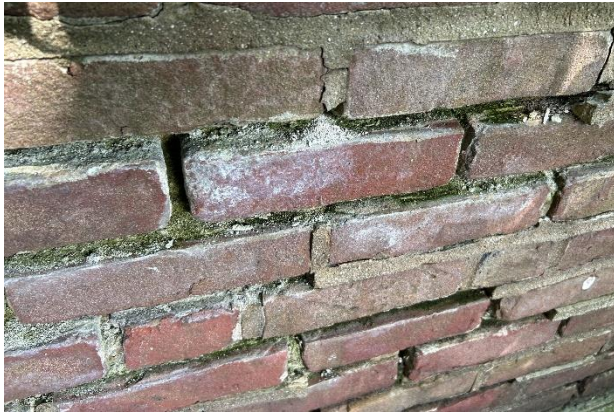
Figure 16. Deteriorated mortar joints and loose bricks.
