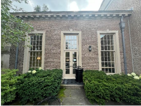
Figure 14. Overview of east courtyard, looking west to entrance wing of library.
