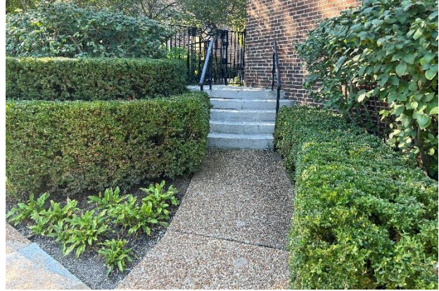
Figure 51. Exit stair and sidewalk from east courtyard.
