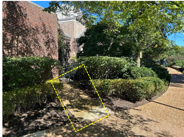
Figure 49. Exit from west courtyard. The portion of the sidewalk from the gate to the main sidewalk will be replaced to accommodate grading changes.
