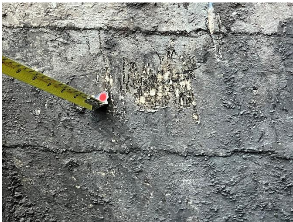
Figure 28. Dampproofing on foundation wall.
