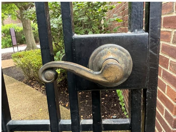
Figure 52. Existing gate hardware.
