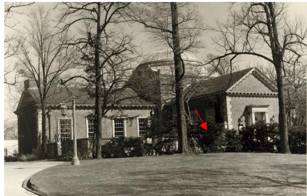
Figure 4. View from the southwest, 1975, showing the reduced height of the garden walls prior to the 1978 additions.
