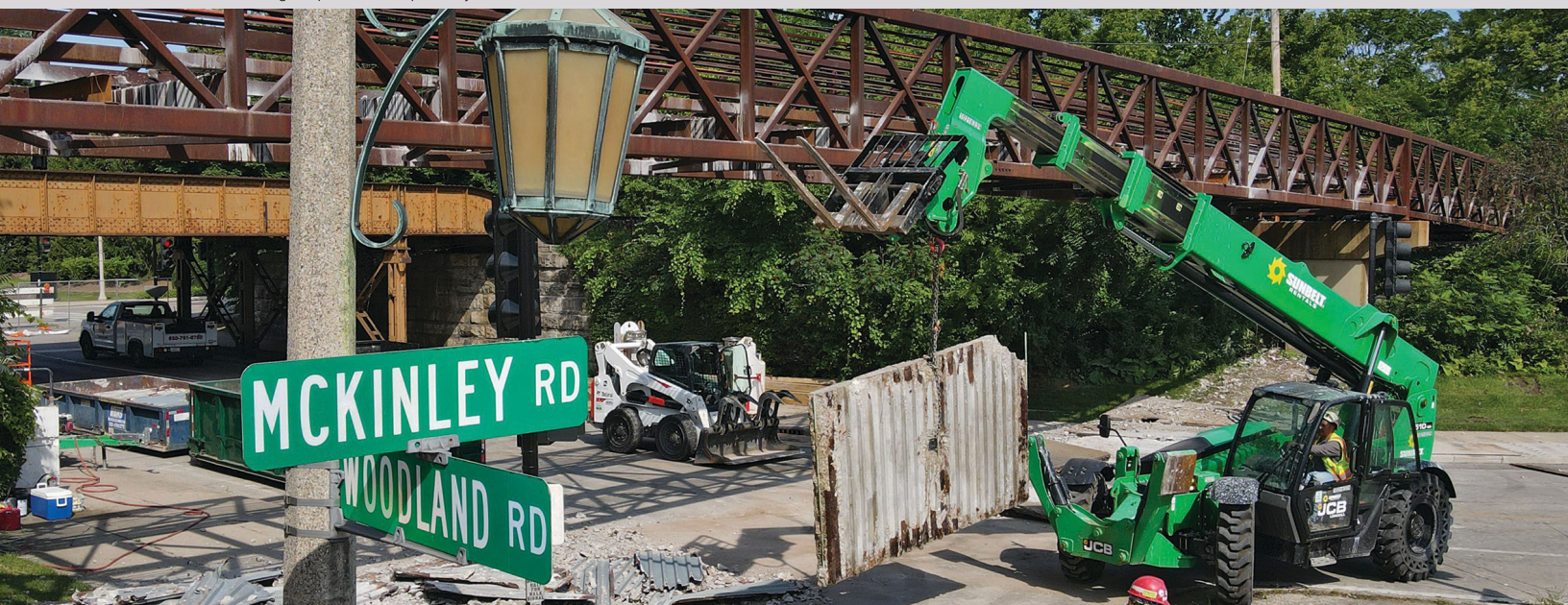
Woodland Pedestrian Bridge Replacement Capital Project
