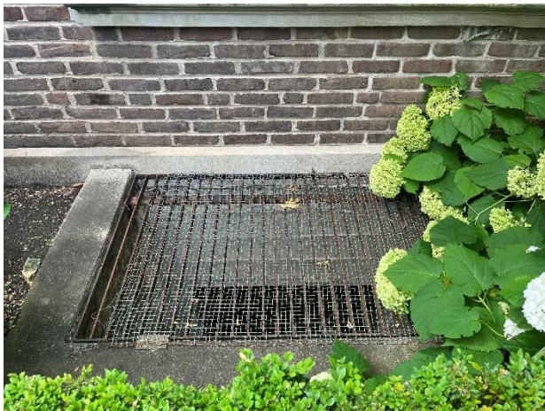
Figure 40. Typical window well.
