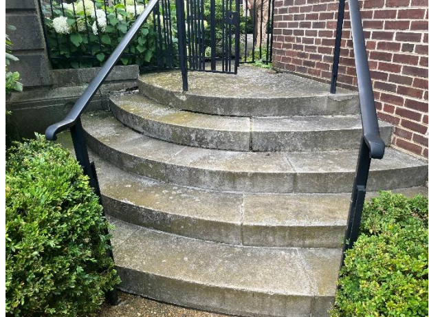
Figure 33. Stairs at the east courtyard gate.
