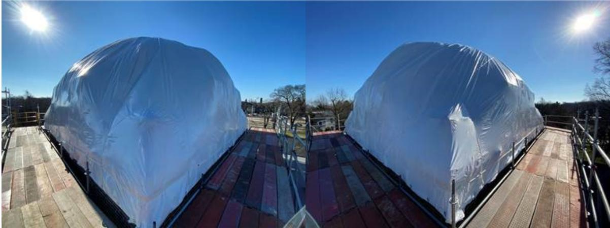
Extra shrink wrap heated and wrapped over sharp corners. This was an area where the previous wrap had started to give out. Belfor cut and adhered extra wrap here to help reduce the time in which the dome will break through the tarp.
