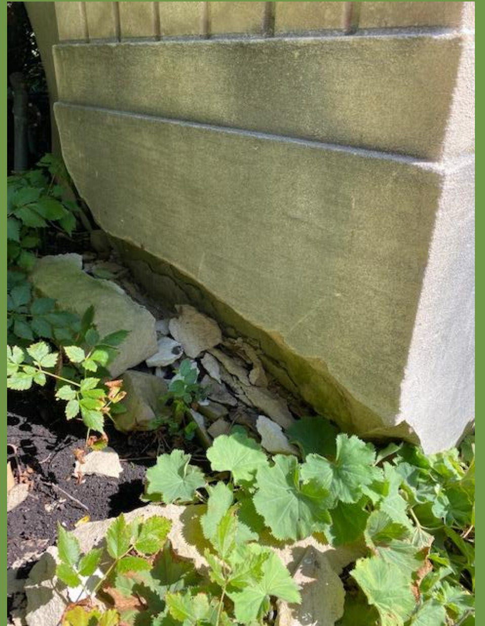
DISCOLORATION + DETERIORATION OF LIMESTONE BASES ON 3 OUT OF 4 PILLARS DUE TO STORMWATER EROSION
