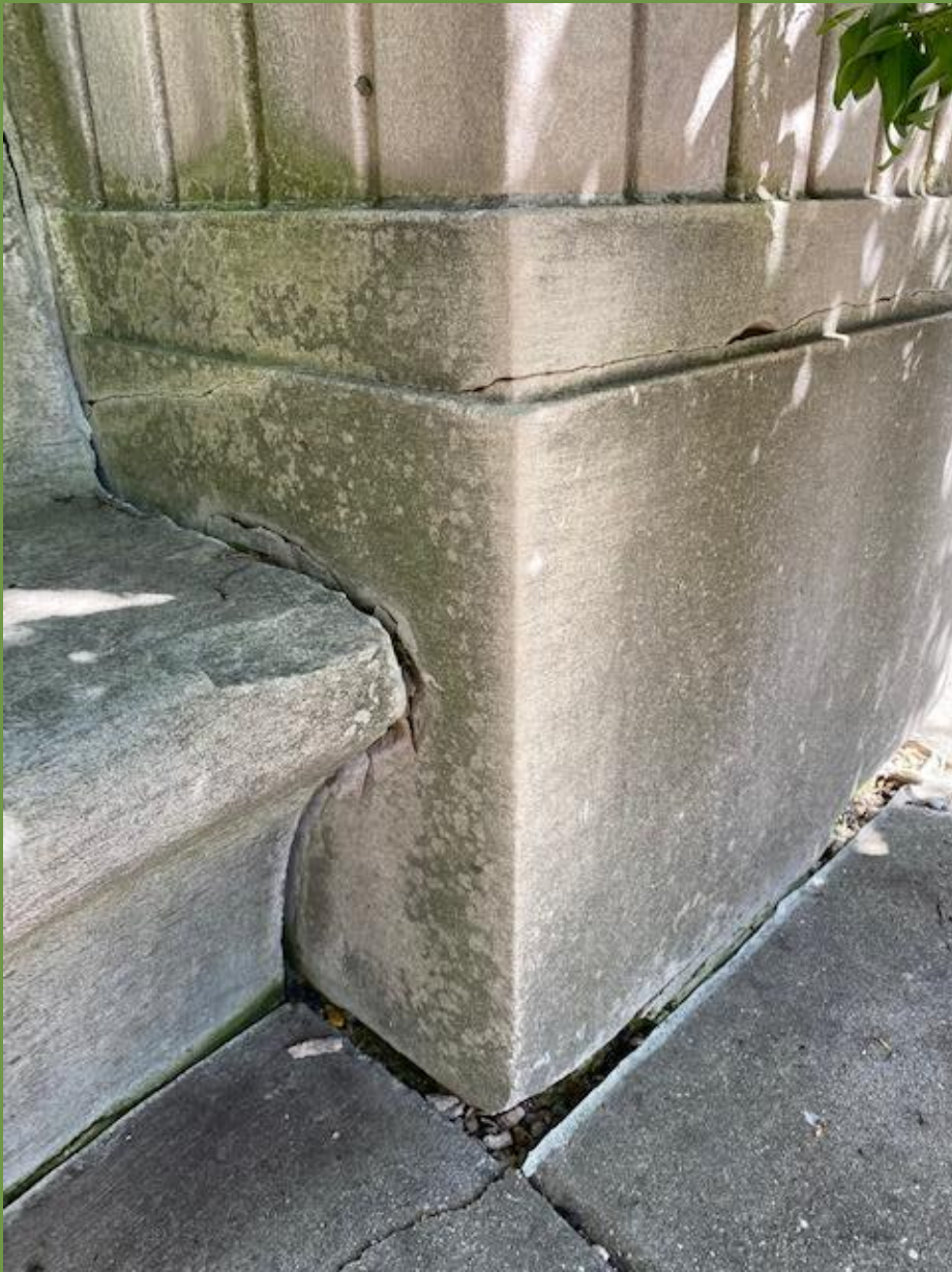
DISCOLORATION + DETERIORATION OF LIMESTONE BASES ON 3 OUT OF 4 PILLARS DUE TO STORMWATER EROSION
