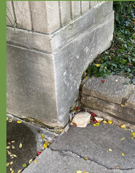
DISCOLORATION + DETERIORATION OF LIMESTONE BASES ON 3 OUT OF 4 PILLARS DUE TO STORMWATER EROSION
