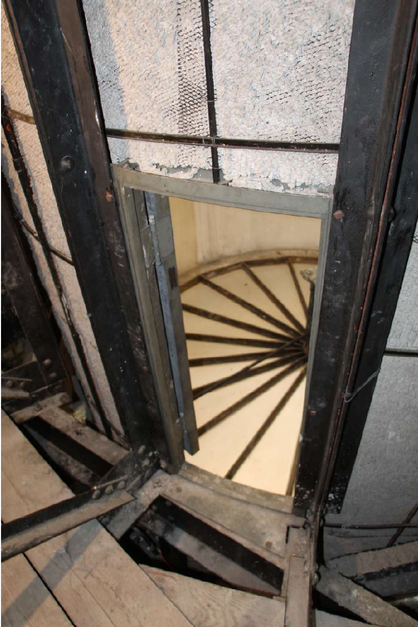
Figure 3. Access door from attic into laylight area.
