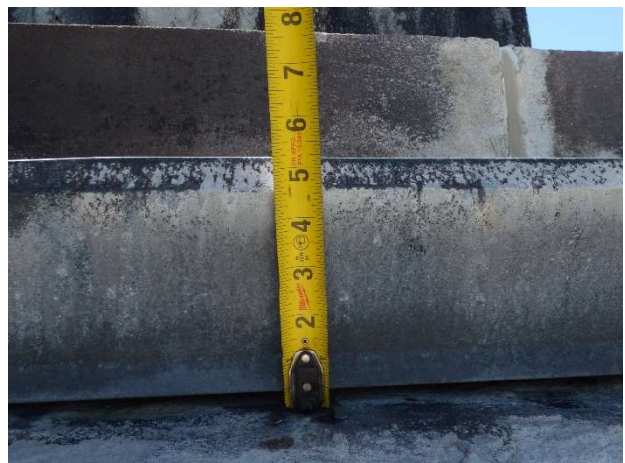
Figure 10. View of gutter at lowest watertable.
