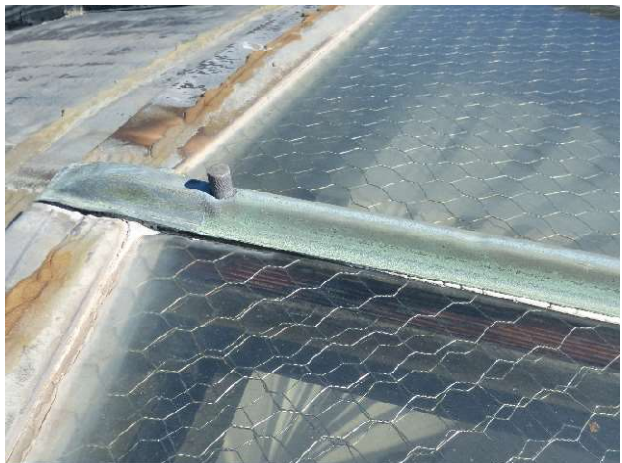
Figure 4. Detail of stop securing skylight glazing.
