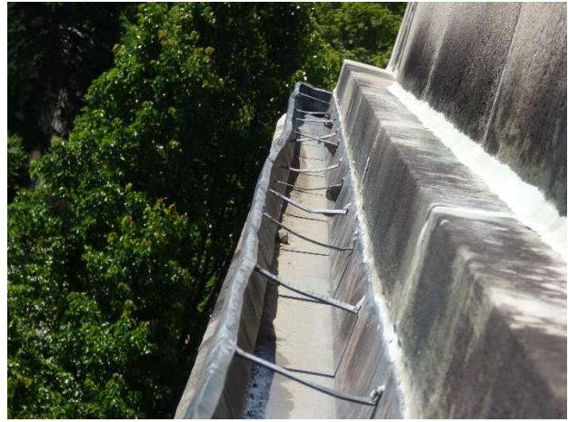
Figure 8. View of gutter at lowest watertable.
