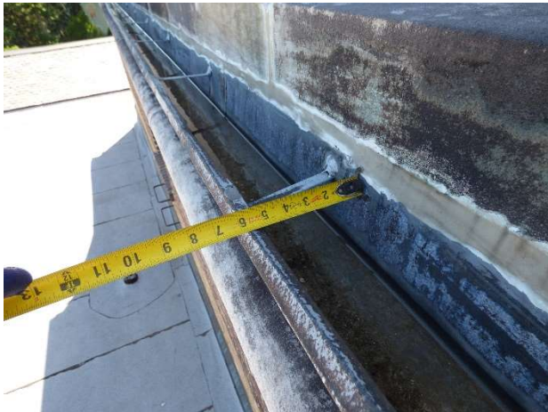
Figure 9. View of gutter at lowest watertable.
