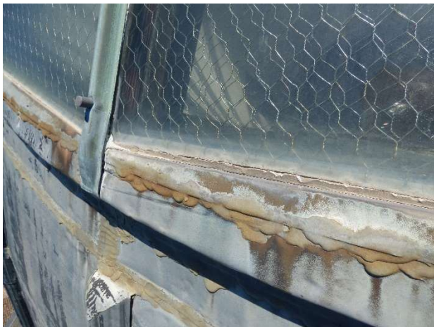
Figure 5. Detail of base of skylight.
