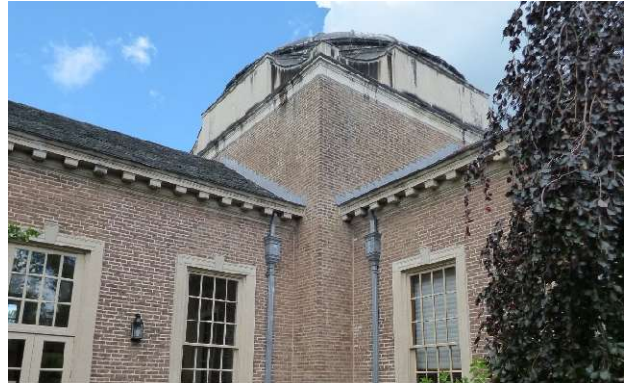
Figure 14. View from the southeast.
